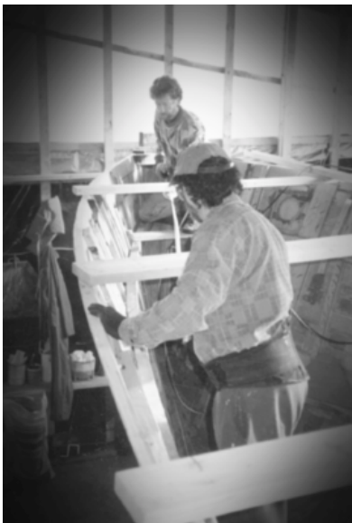
Steamed oak clamps on long horizontal boards to increase rigidity and form.
