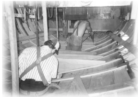
Installing new hull ribs
