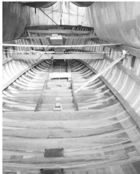
Hull complete with new: ribs, floors, engine bed stringers, and clamps.
